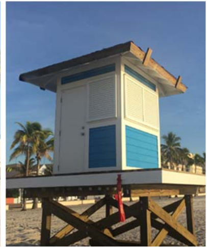
Work in progress, Lifeguard Tower
