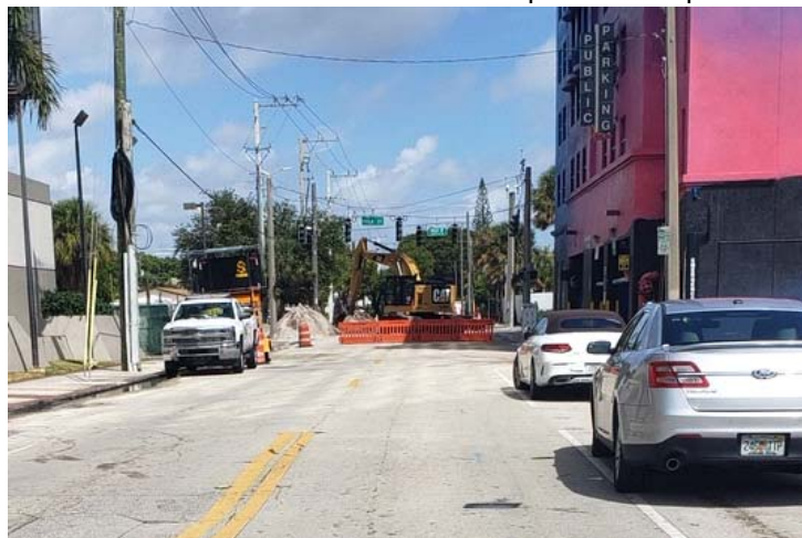
Utility construction at Polk Street and 19 th Avenue
