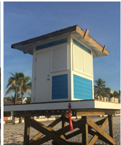
Work in progress, Lifeguard Tower
