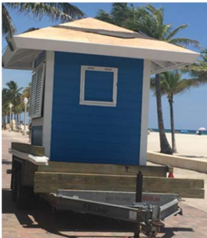
Tower Delivery, Lifeguard Station
