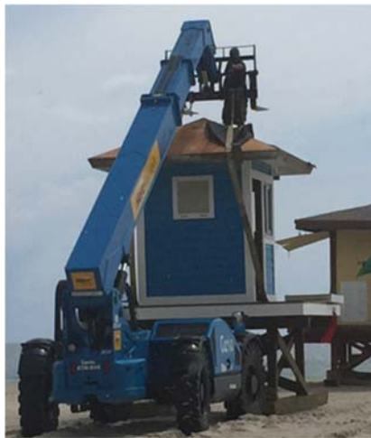
Tower assembly, Lifeguard Tower
