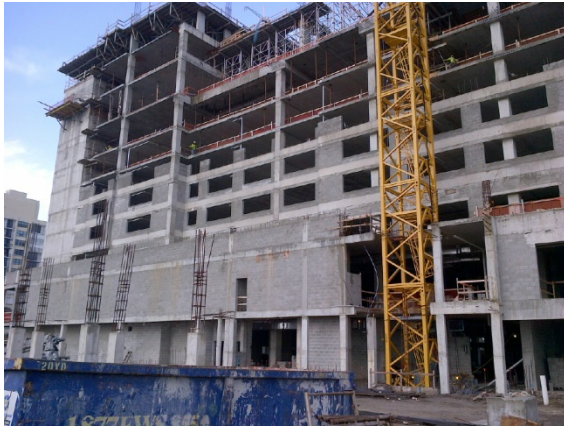
Figure 1: Progress of Concrete Block installation on 6th level
