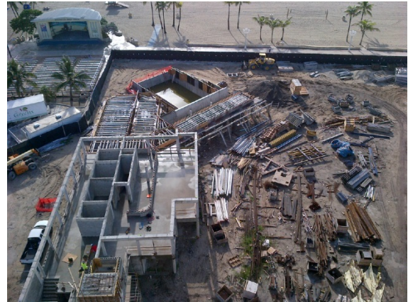
Figure 2: Progress on Landshark Bar
