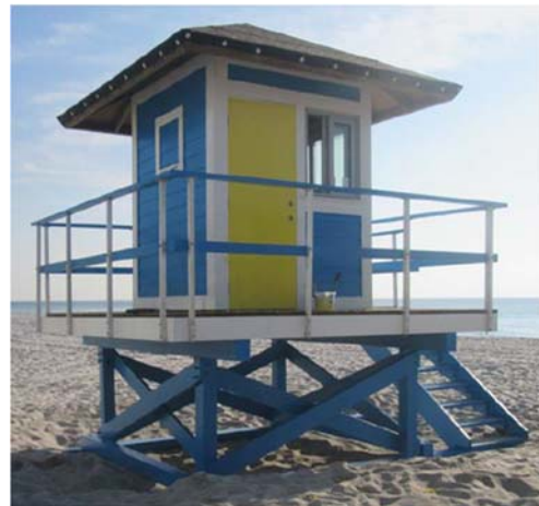
Paint application, Lifeguard Tower
