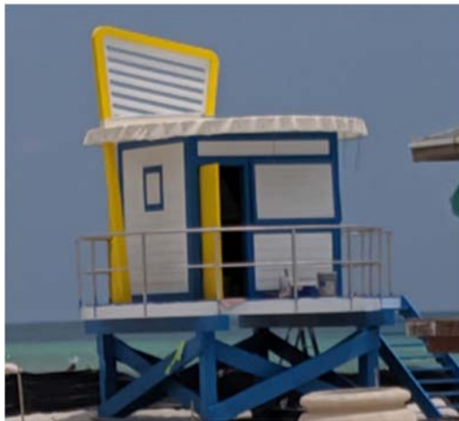
Paint application, First Aid Station
