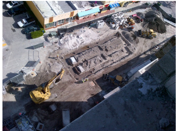
Figure 2: Commencement of public restrooms on Johnson St.
