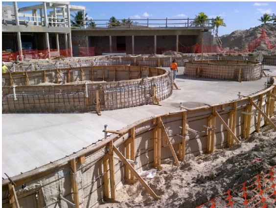
Figure 1: Progress on Family Pool
