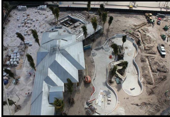
Landshark Bar and adjacent pool progress
