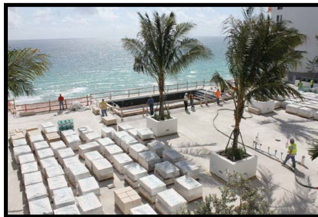
Level 11 pool deck pavers delivered and awaiting installation
